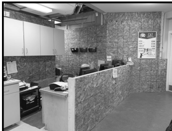
New, temporary customer service area
